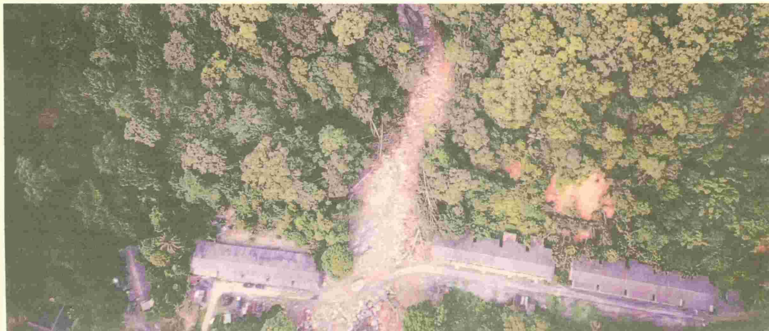
Quarters of the Forestry Department destroyed after heavy rains and mudslides.
